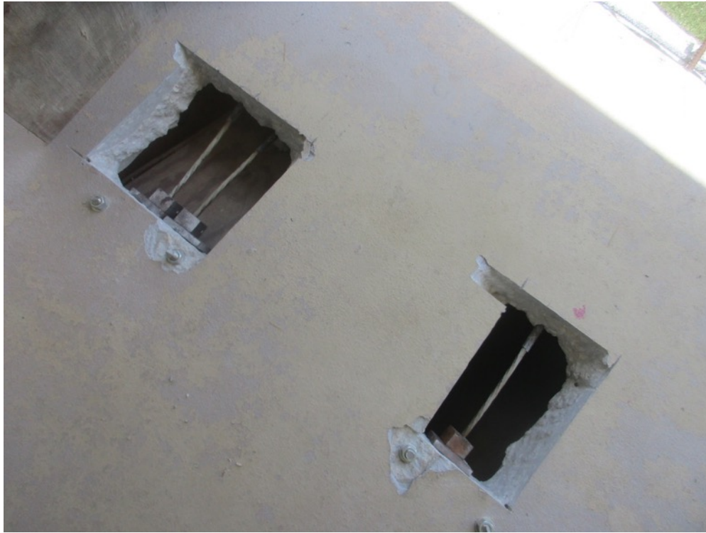
View of east-west PT cables locked-off on the Unit 313 balcony
