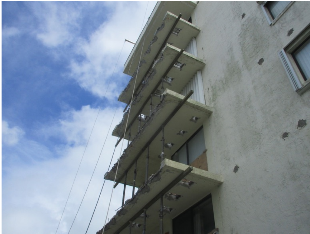
View of PT cable lock-offs installed on the 01 stack north elevation
