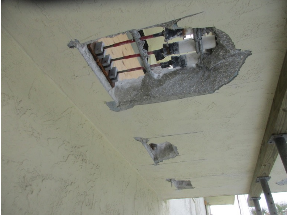
View showing PT cables locked-off on the Unit 111 balcony
