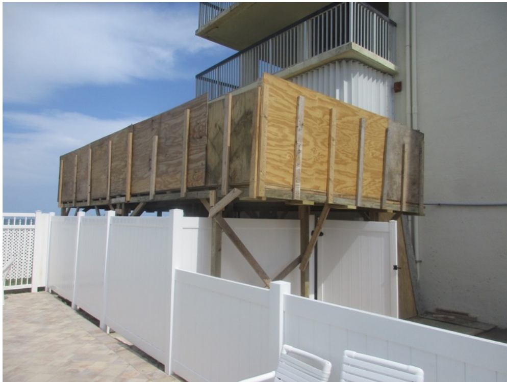
View of pool pump protection constructed on the building 3 northeast corner
