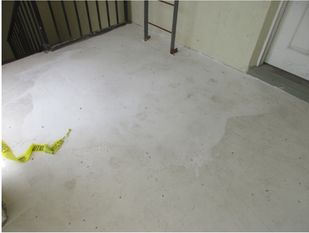
View of final surface profiling completed outside Unit 251 on the walkway
