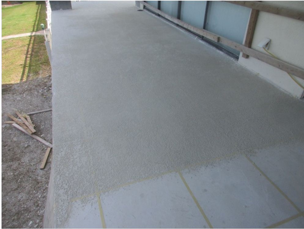
View of knockdown texture application in-progress on the Unit 214 balcony deck
