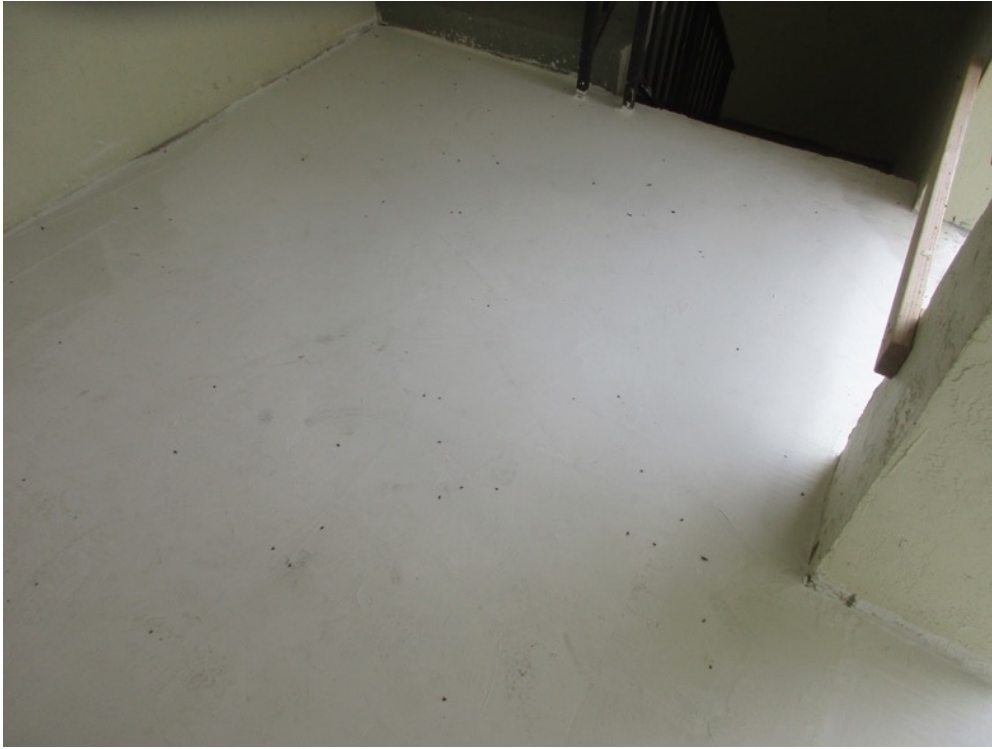
View of final surface profiling completed outside Unit 244 on the walkway
