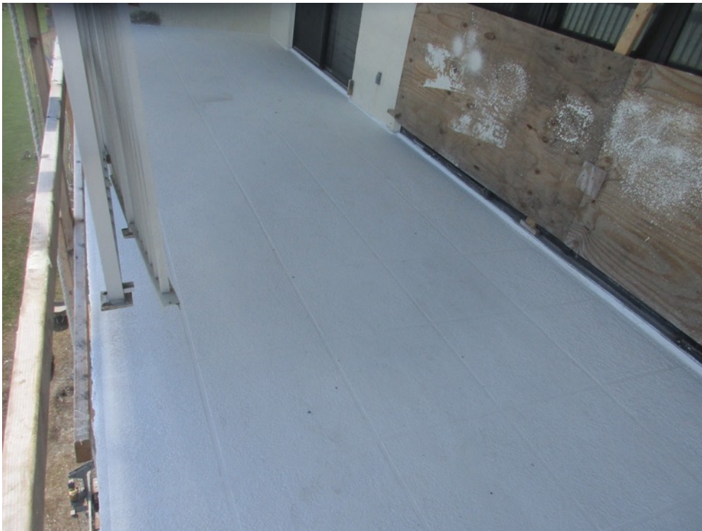
View of tile pattern knockdown texture applied on the Unit 151 east side balcony
