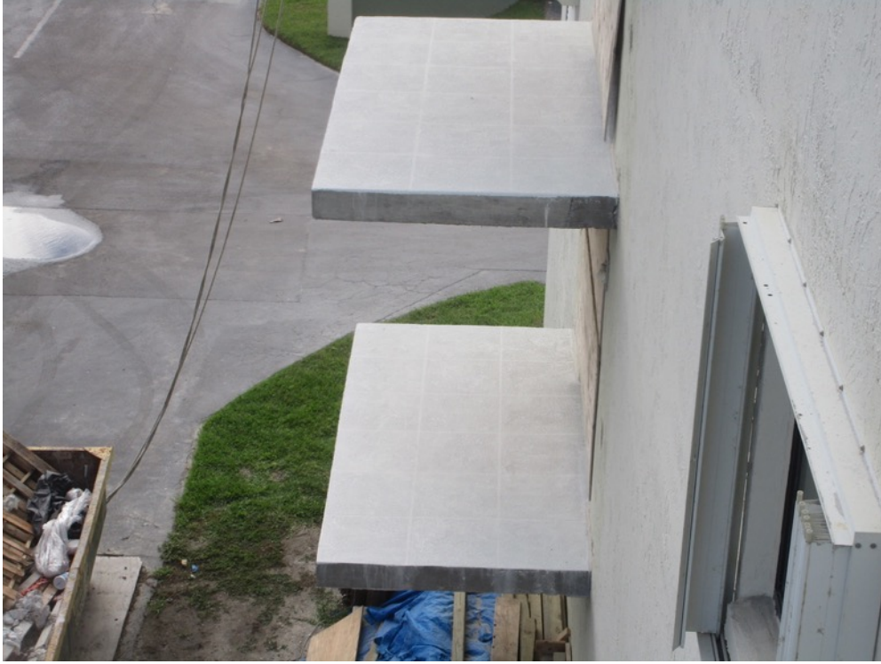
View of tile pattern knockdown texture applied on the Unit 114 and 124 balcony decks
