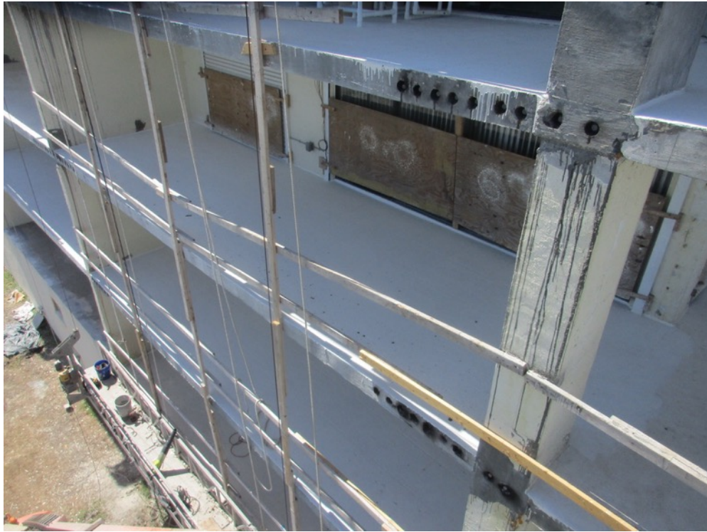
View of tile pattern knockdown texture applied on the Unit 121 and 131 east side balconies
