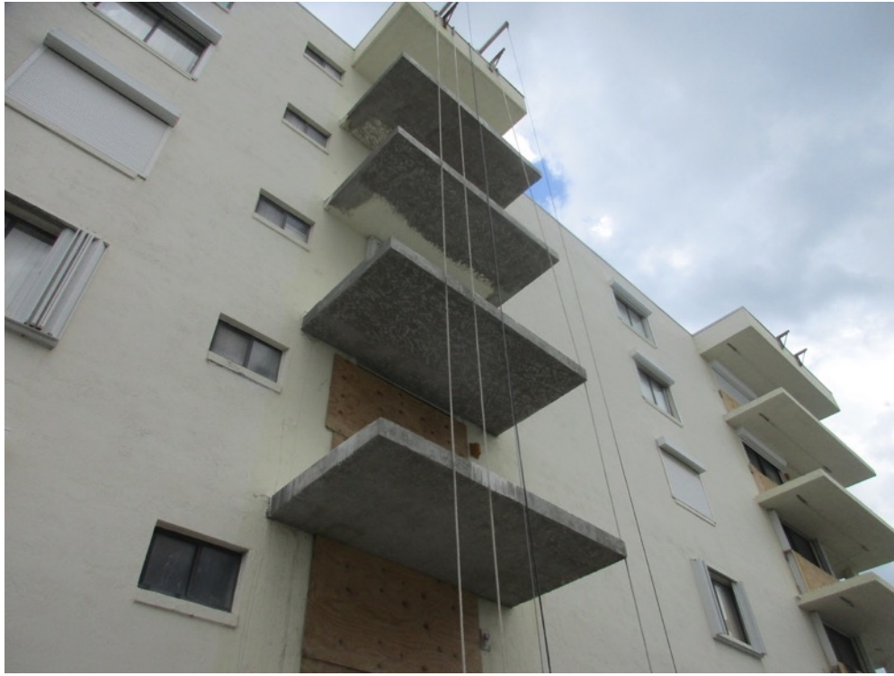
View of stucco finish applied to the 04 stack south side balconies
