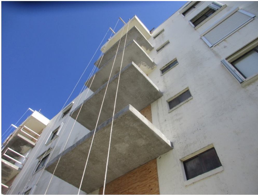
View of stucco finish applied to the 01 stack north side balconies
