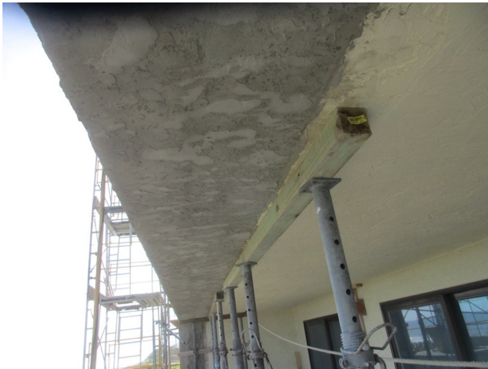
View of stucco finish applied on the Unit 221 slab edge
