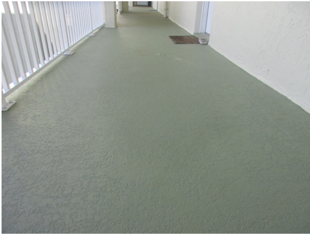
View of deck coats/cut-ins completed on the 401 building 4 th floor walkway
