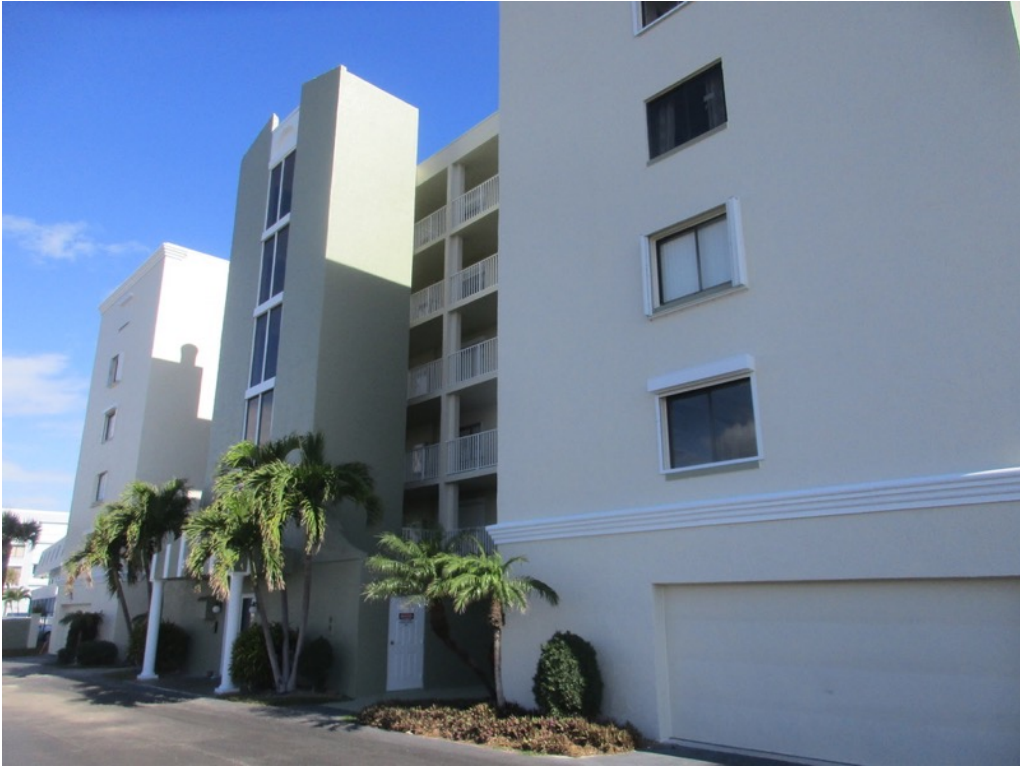
View of coatings applied to the 401 building west elevation
