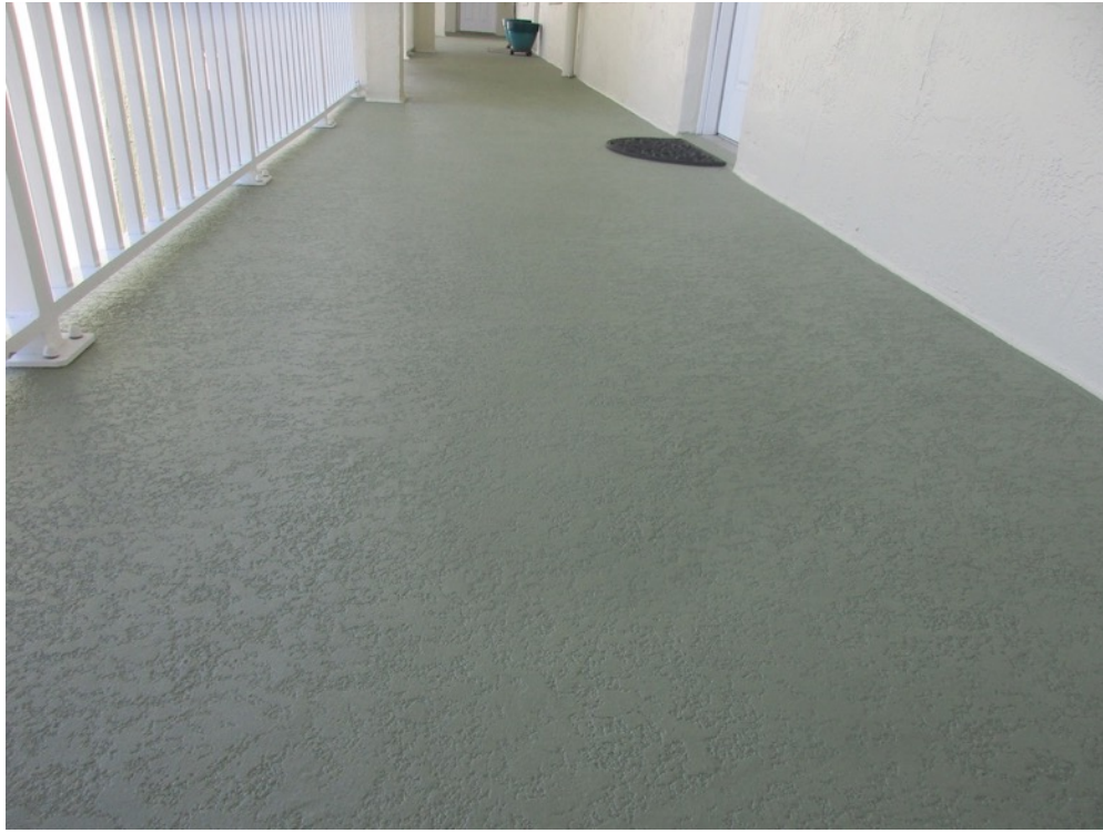
View of deck coats/cut-ins completed on the 401 building 5 th floor walkway
