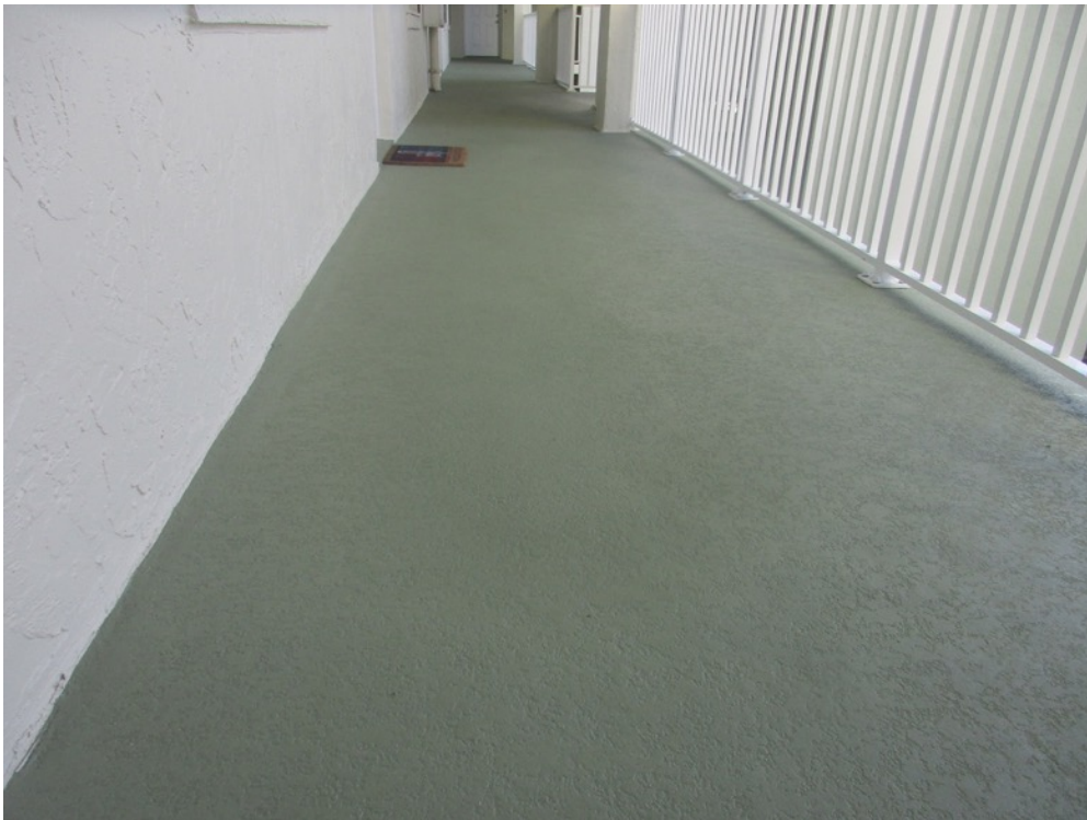
View of deck coats/cut-ins completed on the 401 building 3 rd floor walkway
