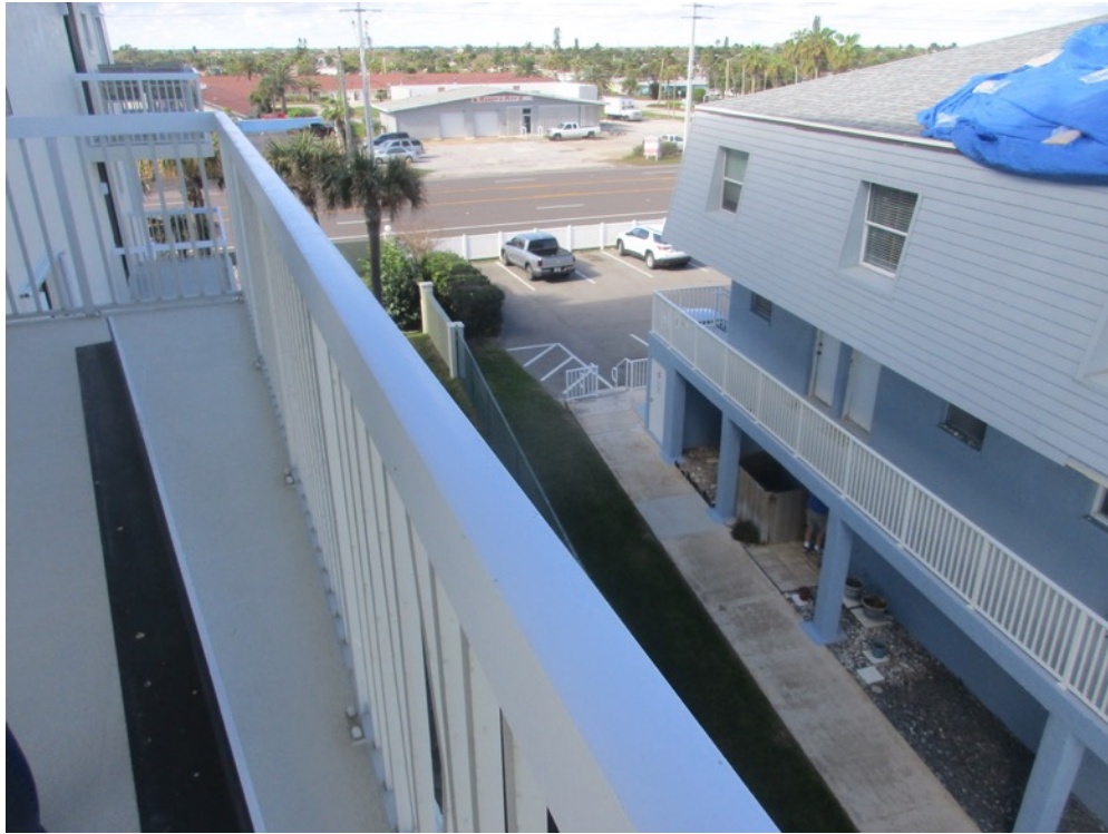
View of handrail top cap painted on the Unit 131 balcony
