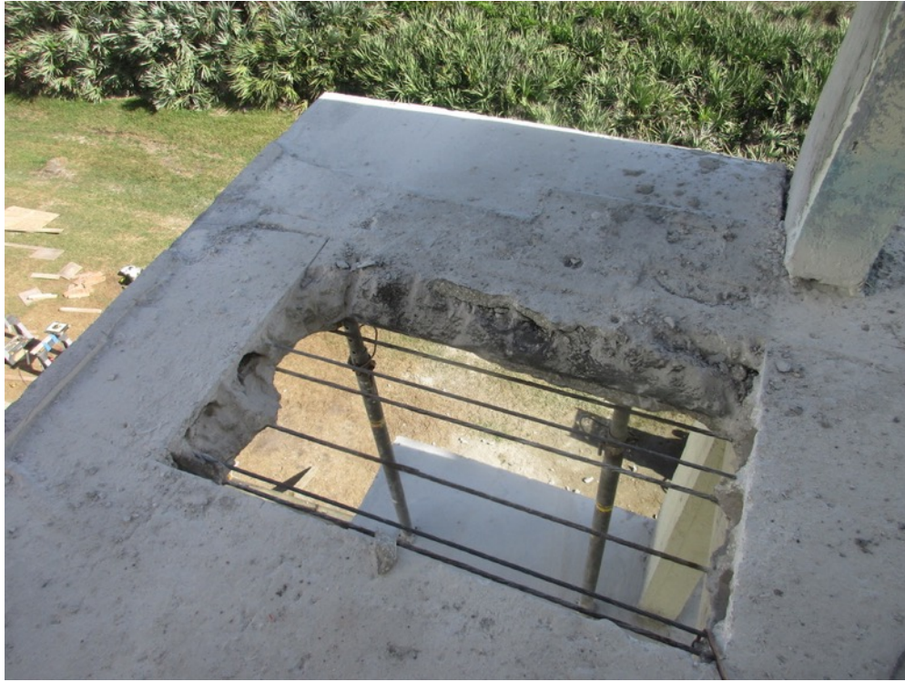
View of full depth/slab edge excavations in-progress on the Unit 231 balcony
