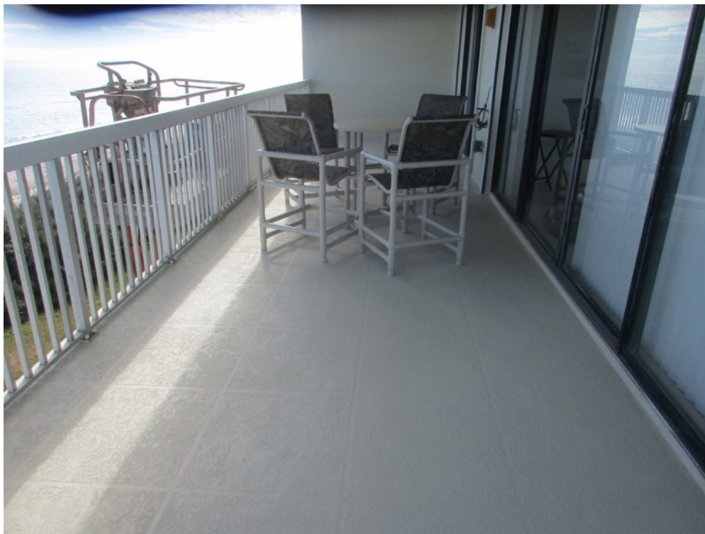
View of deck coatings applied on the Unit 131 balcony
