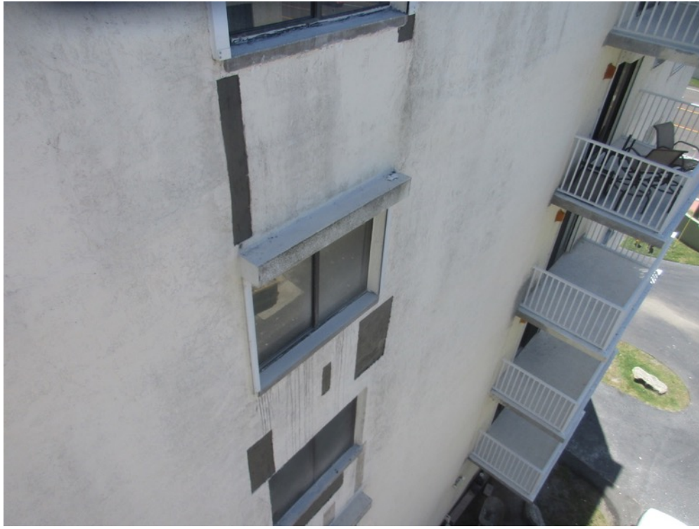
View of delaminated stucco repairs in-progress on the north elevation shearwall
