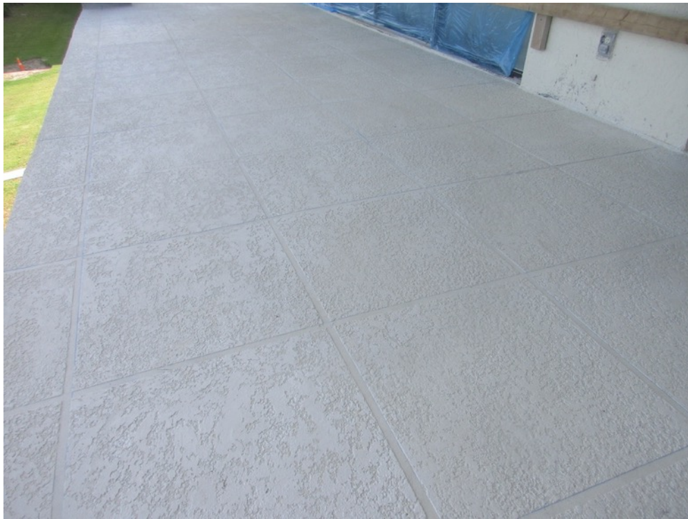
View of knockdown texture applied on the Unit 224 balcony deck
