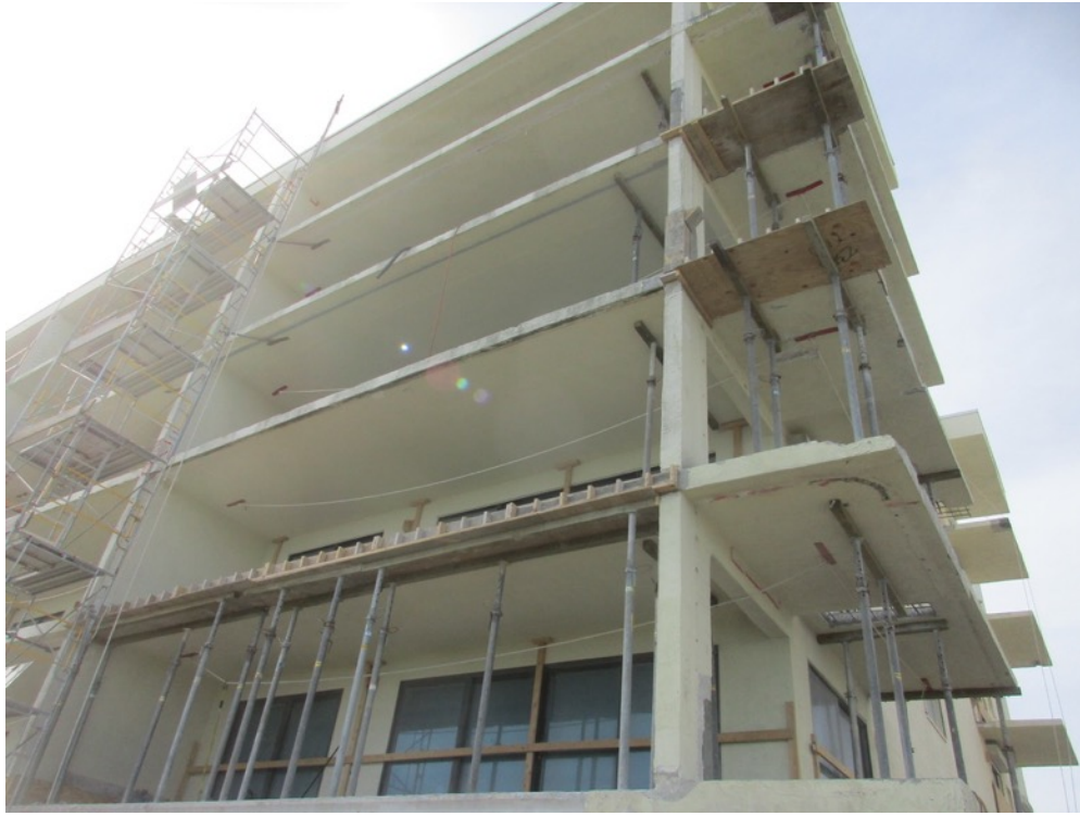
View of form construction in-progress on the 403 building 01 stack
