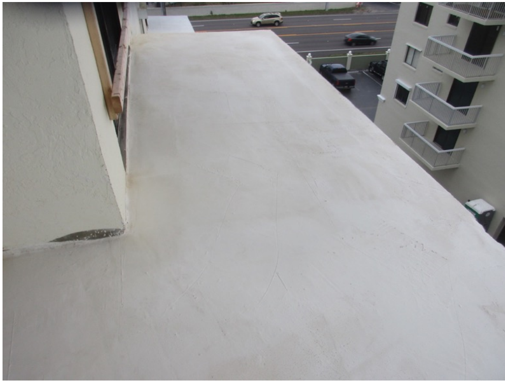
View of skim coat applied on the Unit 251 balcony north elevation
