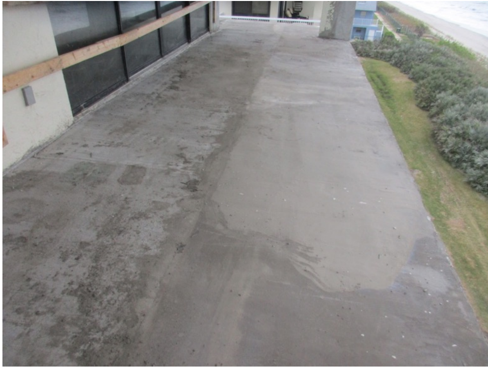
View of topping repairs cast back on the Unit 241 balcony
