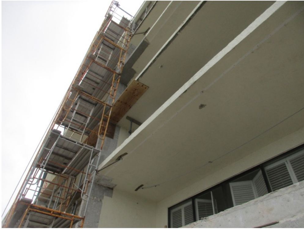
View of column excavations in-progress on the 03/04 balcony stack divider walls
