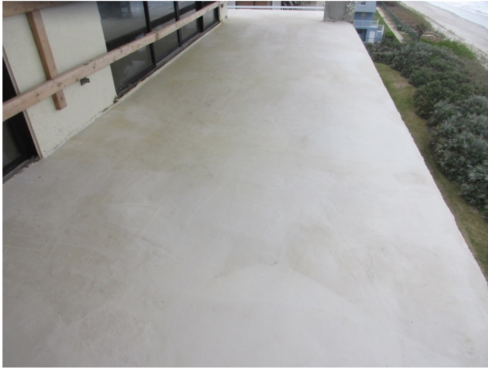
View of skim coat applied on the Unit 251 balcony east elevation
