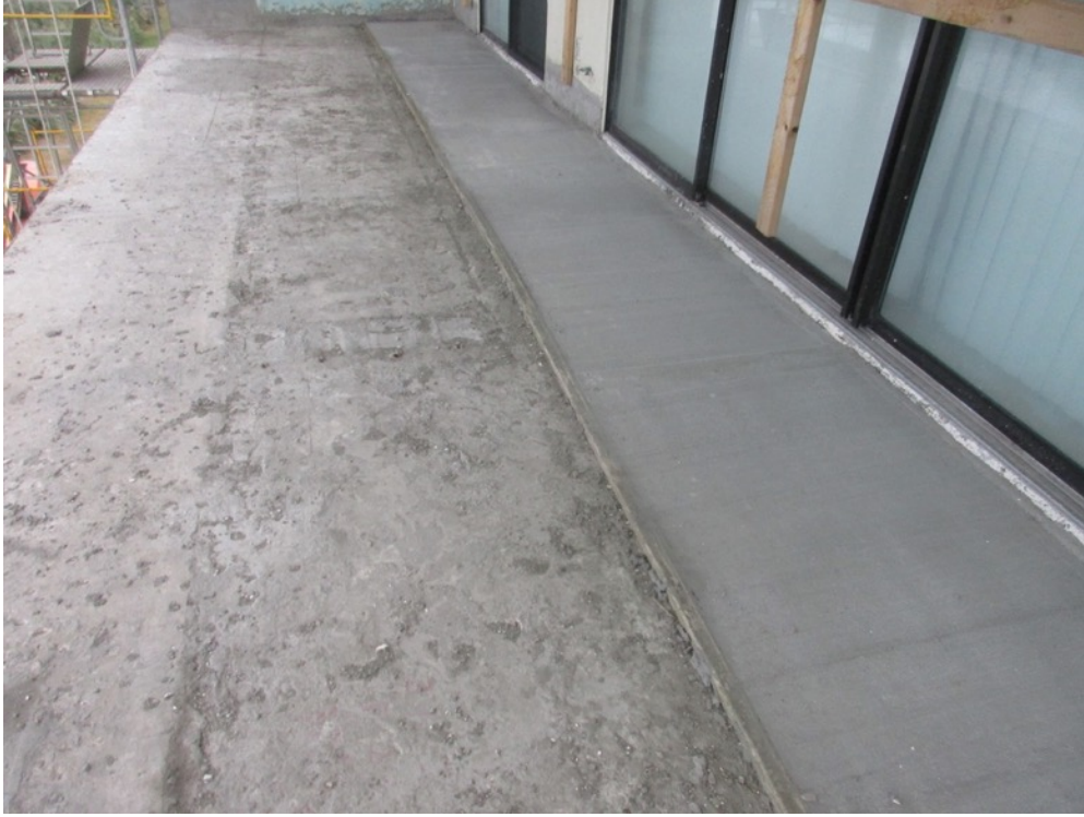
View of topping casting in-progress on the Unit 231 balcony
