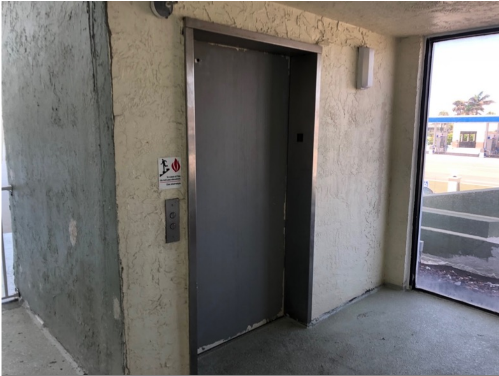
View of surface prep in-progress on the 1 st floor elevator door
