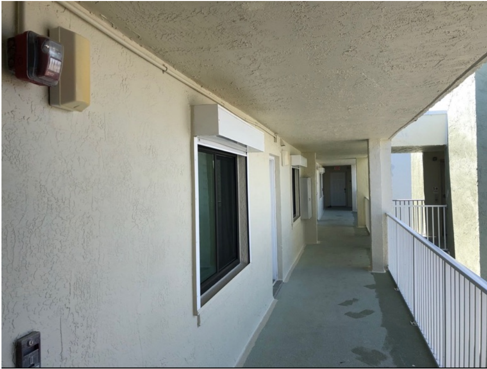
View of wall/ceiling coatings applied on the 6 th floor walkway
