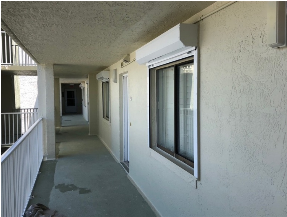
View of wall/ceiling coatings applied on the 5 th floor walkway
