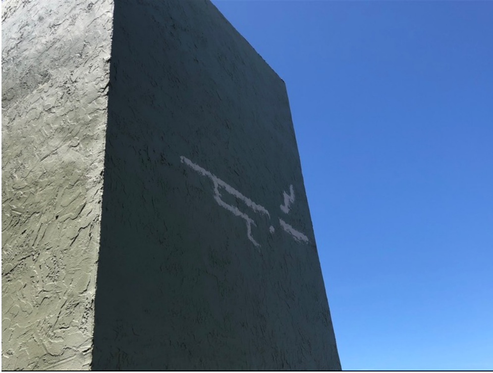
View of elastomeric crack treatment on the elevator tower
